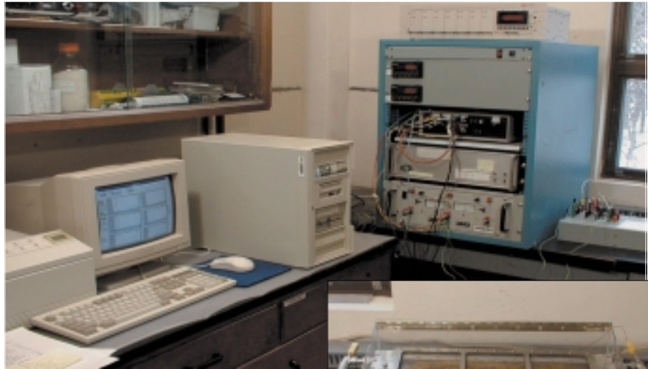
Voltage control and data-logging section
