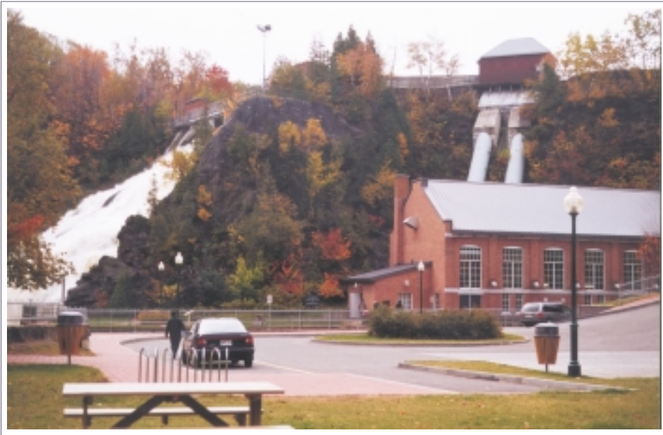
Riviere du Loup Small Hydro Plant
