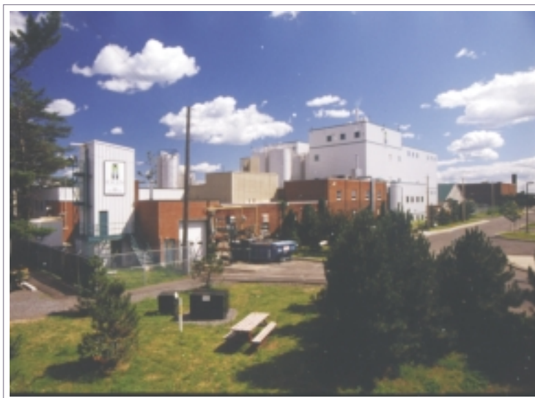
Iogen Corporation's Biomass Ethanol Plant
