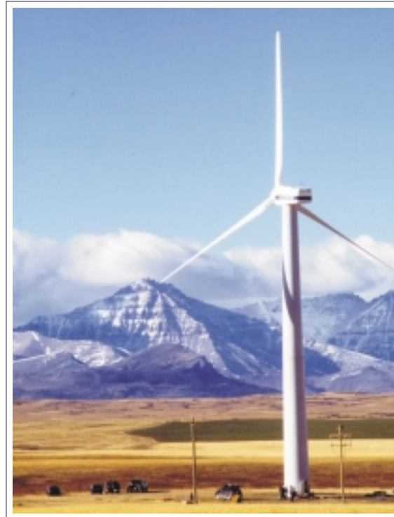
660 kW Vestas Wind Turbine in southern Alberta - Four such turbines supply green power to customers in Calgary (Photo courtesy of Vision Quest Windelectric Inc.)
