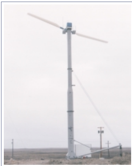
80-kW Wind Turbine, Cambridge Bay, NWT - Courtesy of KHJ Photography/ Kevin Johnston
