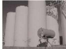
DOUBLE WALL TANKS - 110% CONTAINED
