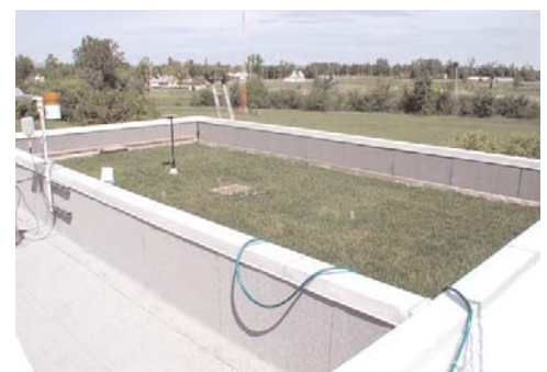
NRC's Field Roofing Facility
