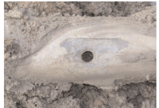
Service connection pull out
