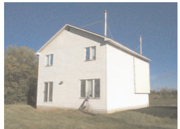
NRC Two-Storey Research House – back
