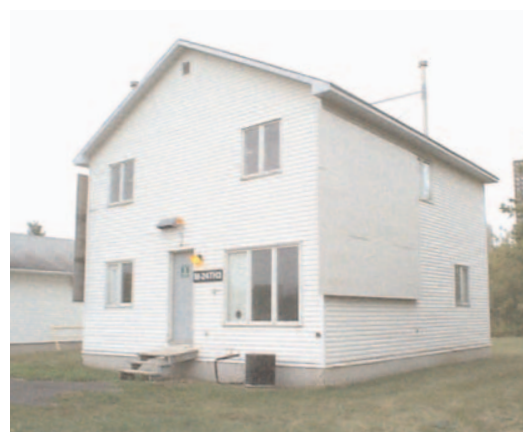
NRC Two-Storey Research House – front
