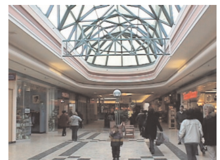
Skylights can enhance a building if properly designed and installed
