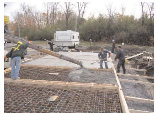
Preparation of test slabs on the NRC campus.
