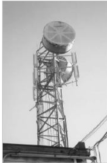
Figure 8. Cell site with microwave link
