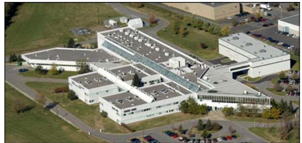
NRC-IMI's facilities in Boucherville including the new prototyping and incubation facilities
