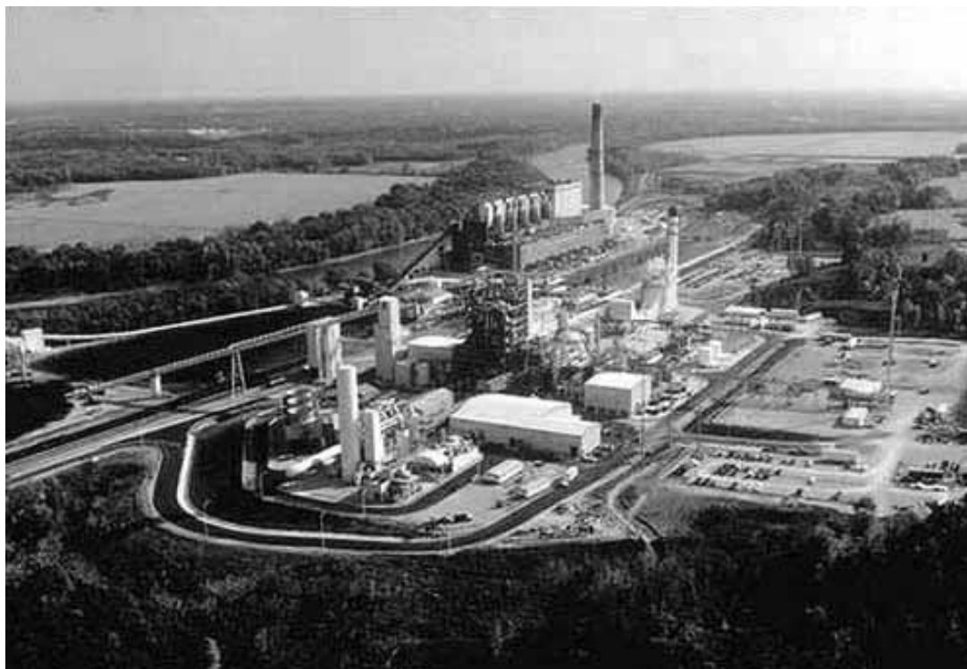
The Wabash River Integrated Gasification Combined-Cycle Plant, Indiana, U.S.A.
