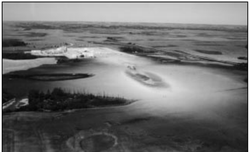
Figure 2.2 SCC pipeline failure site: Rapid City, Manitoba, July 1995
