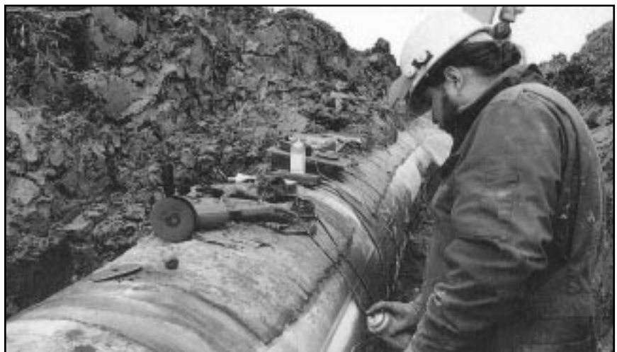
Figure 4.5 Magnetic particle inspection
