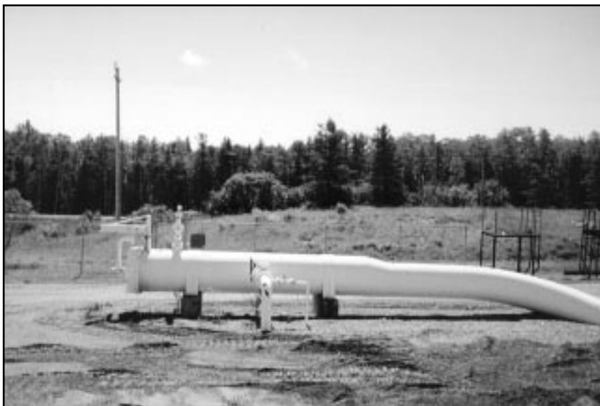
Figure 4.8 Pig receiver
