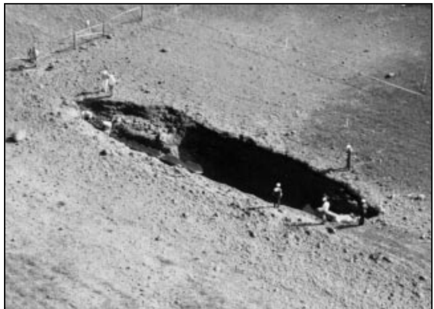
Figure 5.2 Pipeline failure site: Williamstown, Ontario, October 1994
