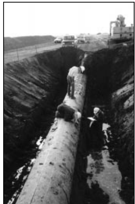
Figure 4.4 Investigative excavation
