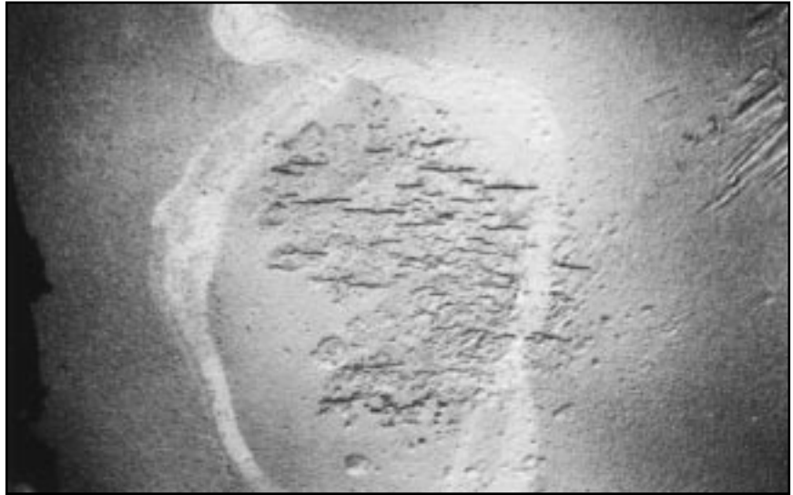
Figure 3.8 Colony of SCC cracks
