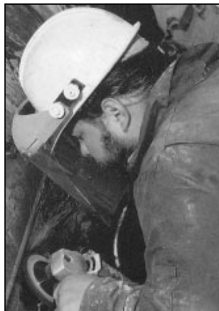
Figure 4.6 Grinding out SCC
