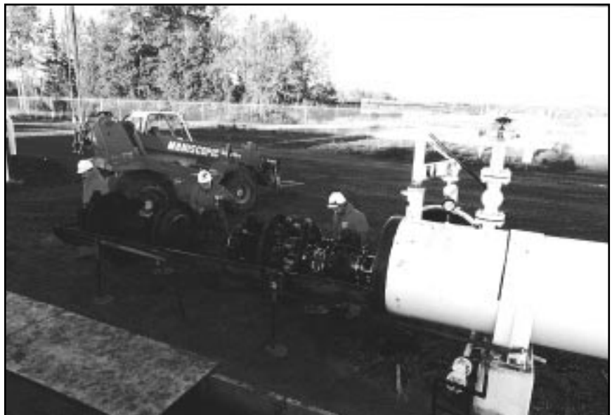
Figure 4.9 British Gas SCC pig being removed from a receiver
