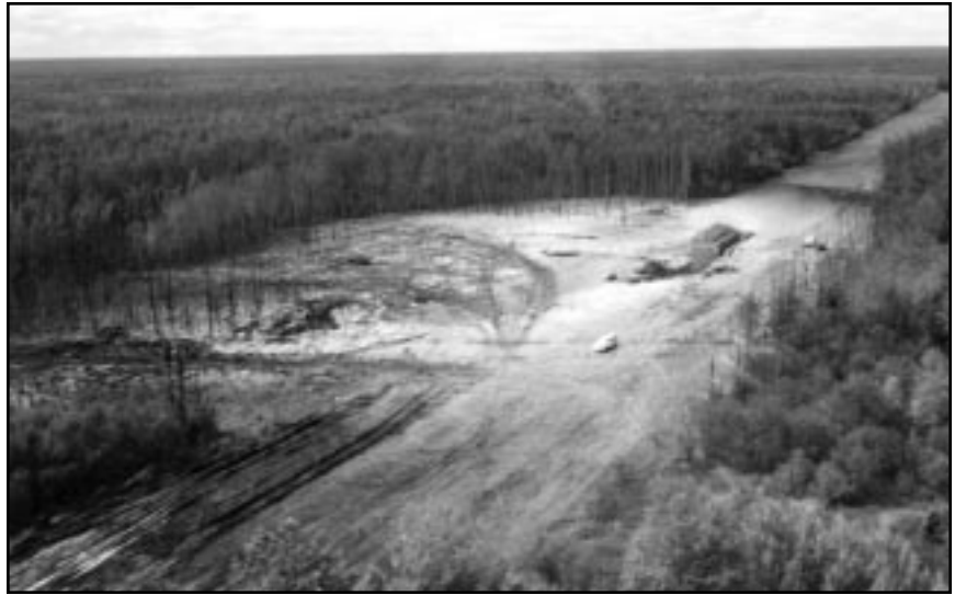
Figure 2.1 SCC pipeline failure site: Lowther, Ontario, August 1985
