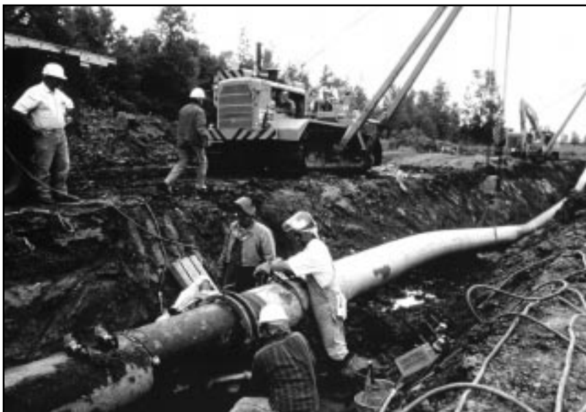
Figure 4.15 Selective pipe replacement
