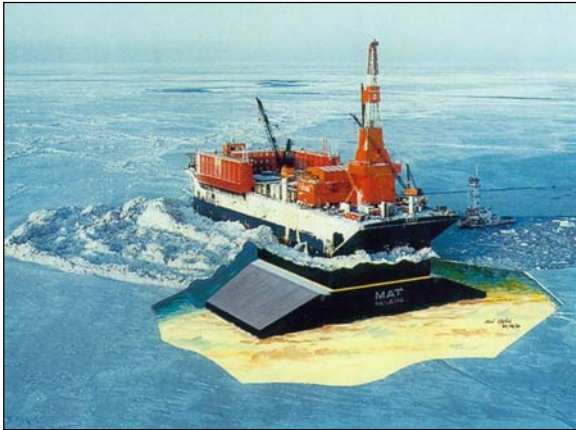
Steel Drilling Caisson
