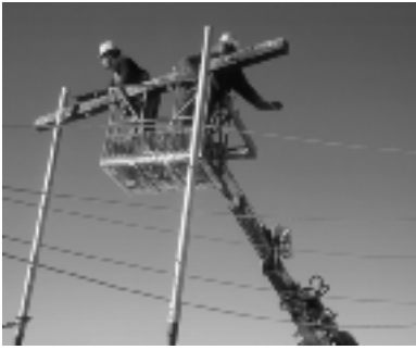
Workers install the transmission line.
