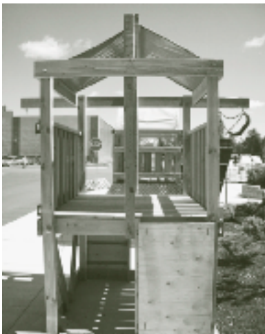
Children could be exposed to arsenic and chromium leaching from playground structures constructed out of CCA pressure-treated wood.
