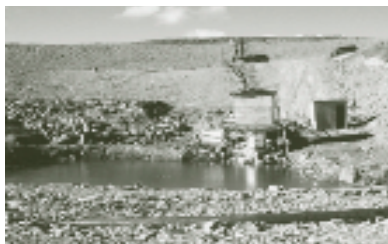
Seepage collection pond at the Mount Nansen Mine
