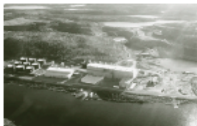
Colomac mine site from the air Large fuel storage containers (left) are leaking into the lake. Heavy equipment and hazardous materials have been abandoned at the mine site.
