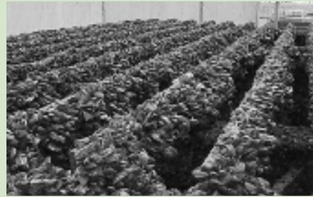
De-fouling of water intakes and other equipment infested with zebra mussels, such as these debris racks, cost millions of dollars each year.
