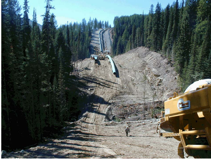
Photo 3-2 Pipeline – Laying
