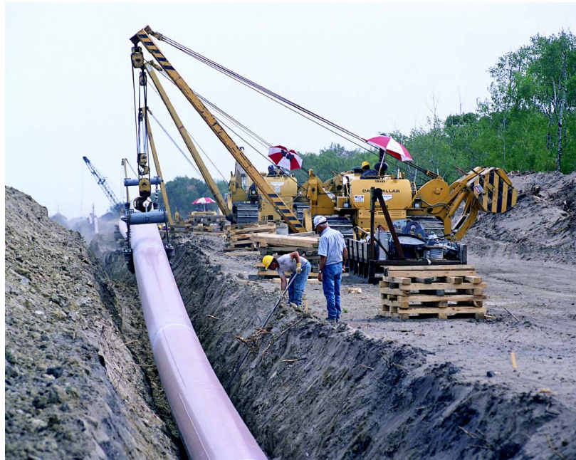
Photo 3-3 Typical Pipeline Construction – Lowering
