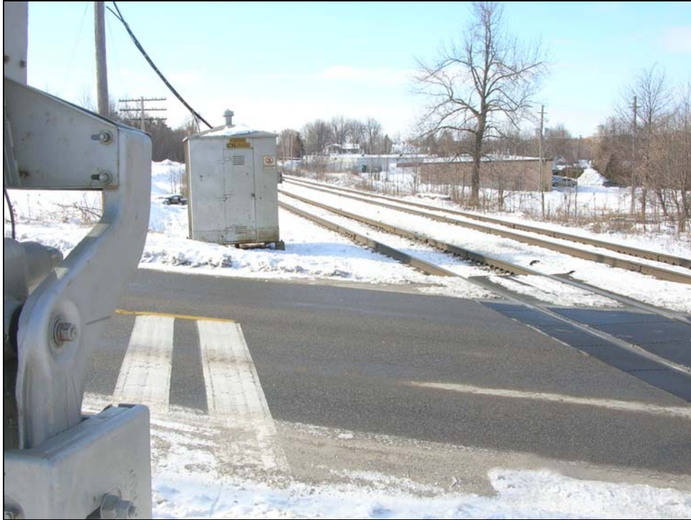
Photo 1. View looking west from sidewalk in southeast quadrant of the Bartholomew Street level crossing
