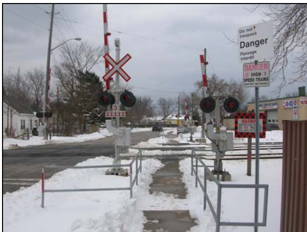
Photo 4. Pedestrian gate installation at Alexandra Road crossing at grade along the Oakville Subdivision in Mississauga, Ontario
