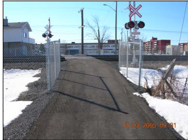
Photo 3. Pedestrian only crossing near school in Kingston, Ontario
