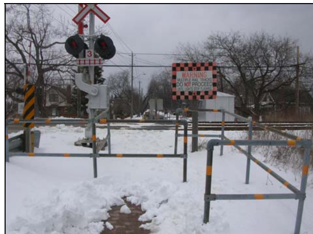
Photo 5. Pedestrian maze gates installation along the Oakville Subdivision in Mississauga, Ontario
