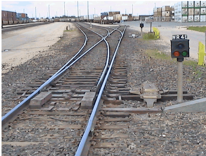
Photo 1. View looking westward into classification tracks at switch WR4E, Symington Yard (TSB photo). Switch aligned for movement into track WI03.
