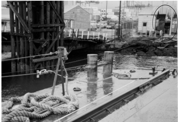
Figure 5 - Starboard quarter of the barge. Mooring winch and lamp post ashore are circled.
