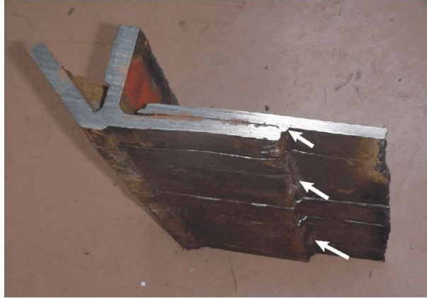
Photo 6. Undamaged end of platform showing weld that connects the underside of the well floor shear plate to the steel angle
