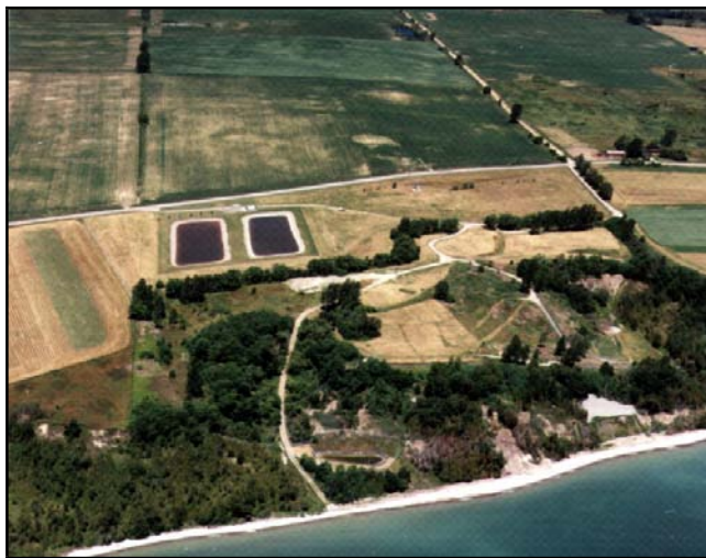
Figure 8.10 – Existing Port Granby Waste Management Facility
