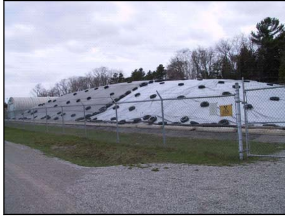
Figure 8.11 – Pine Street Extension Temporary Storage Site
