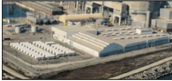
Figure 5.1 PWMF with RCSA on left and Used Fuel Dry Storage Area on right
