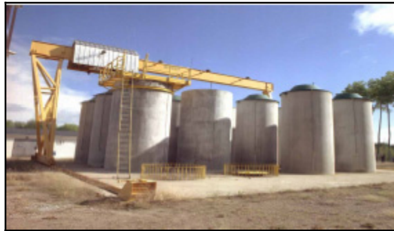
Figure 4.2 AECL Concrete Canisters
