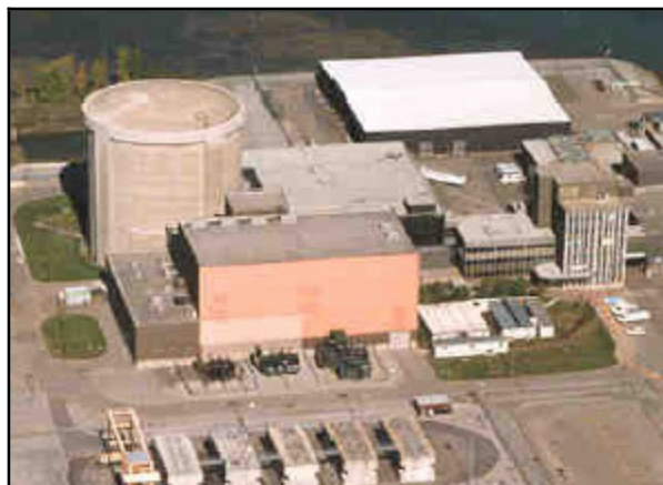
Figure 5.5 Gentilly-1 Waste Management Facility
