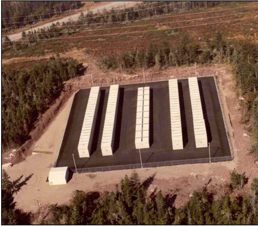
Figure 5.4 SRWMF at Point Lepreau
