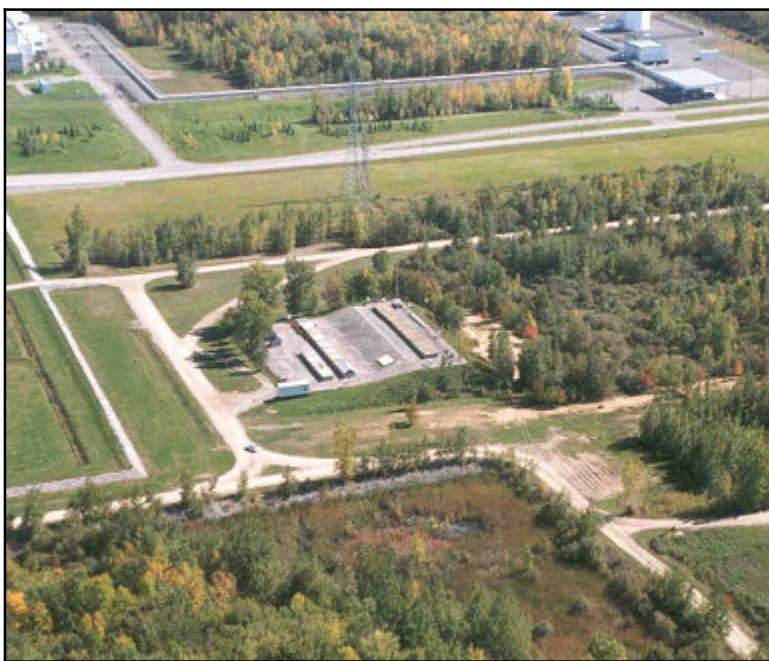
Figure 5.3 Hydro Québec Waste Management Facility
