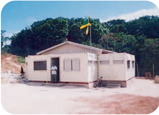
The Mandeville School in Jamaica, made from four shipping containers.
