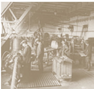
Building the R.100 at Howden
