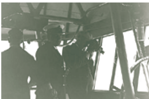
Inside the control car
