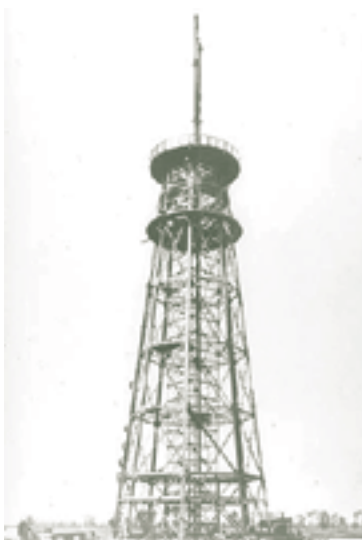
The mooring mast of St Hubert under construction
