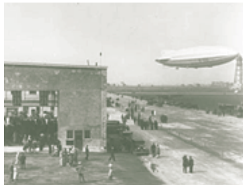
The press hangar at St Hubert
