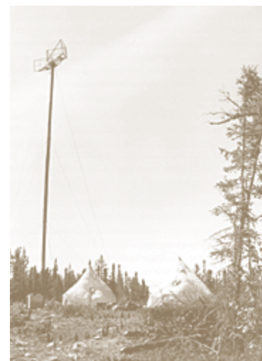
SHORAN camp and antennae, 1950. These ground stations sent radio signals, which were received by the aircraft as part of a radio navigation system that accurately placed the aircraft over the terrain to be photographed. (Public Archives of Canada PA 66363)
