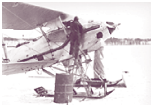
The Test Flight experimented with a number of aircraft in the 1930s; investigative work included the analysis of oil dilution systems for winter starting and aircraft de-icing equipment. This photograph shows personnel refueling a Hawker Audax during winter trials at Rockcliffe in 1934. (Public Archives of Canada PA 62978)
