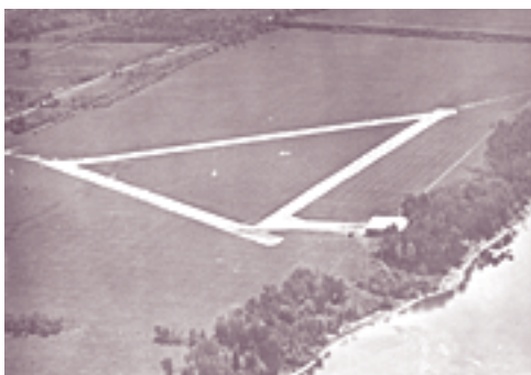
Taken in June 1921, looking southwest, this is the earliest known photograph of Rockcliffe's aerodrome. Established by the Air Board as Ottawa Air Station, a small dock had been installed behind the hangar and a Curtiss HS-2L flying boat was tied up there. The small triangle in the centre of the runways was a code mark indicating a commercial air harbour. (Public Archives of Canada PA 62456)
