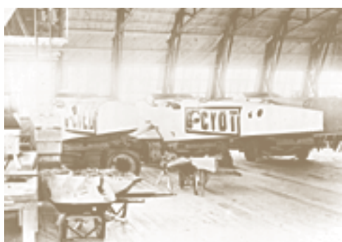
Interior view of the wooden hangar and hull of Curtiss HS-2L flying boat, Rockcliffe, 1922. (Public Archives of Canada PA 62292)
