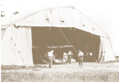
The first hangar at Rockcliffe, photographed in 1921. This is one of the canvas-covered Bessonneau hangars donated by Britain to Canada in 1920. A Bristol F.2B fighter is in the doorway. (Public Archives of Canada RE 18027)
