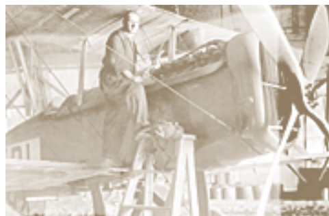
Engine fitter servicing a de Havilland DH-4B of the Canadian Air Board, Rockcliffe, 1921. (Public Archives of Canada PA 117850)
