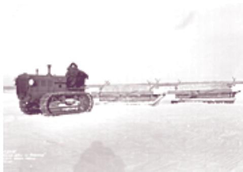
Station maintenance included rolling snow on airfield runways for winter operations, January 1940. (Public Archives of Canada PA 63652)
