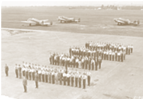
RCAF Station Rockcliffe moved into its wartime operation with an increase in personnel, buildings and units. Here, recruits form into flights near Lockheed Hudson I aircraft of No. 11 (BR) Squadron in September 1939. (Public Archives of Canada PA 63473)
