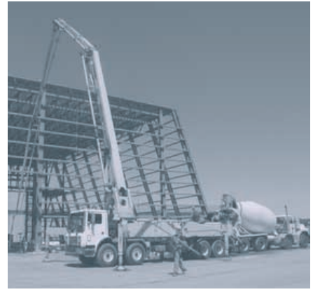
Concrete being poured for the flooring of the new hangar.
