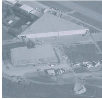
Aerial View of the construction of the Aviation Hangar.
