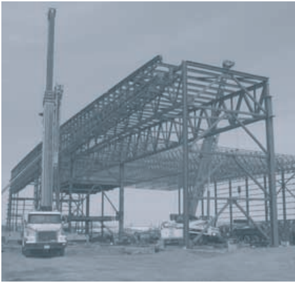
South-west view of the construction of the new hangar.
