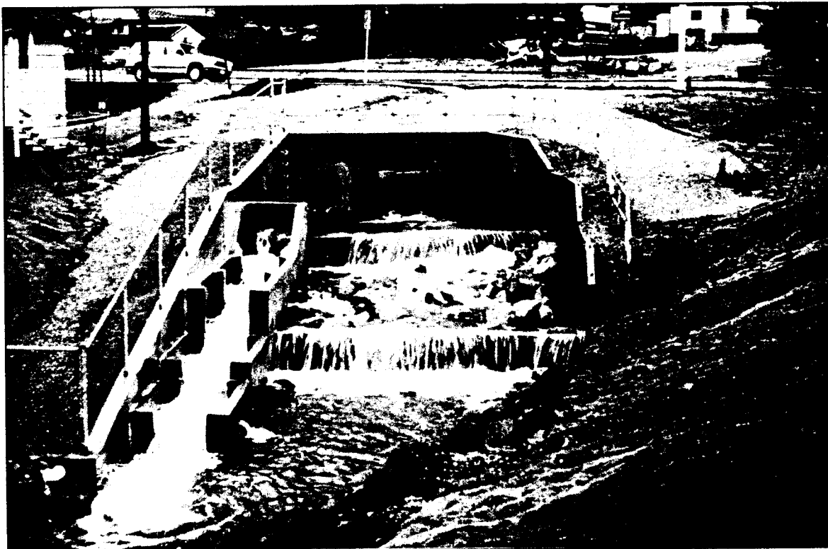
Figure 6.2 Culvert Providing Upstream Fish Passage
