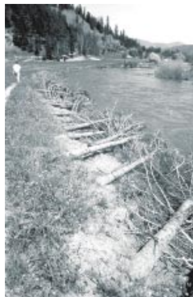
Restoring fish habitat includes placing stumps or branches to shelter juvenile fish from predators.
