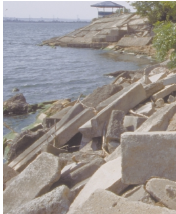
Uncrushed concrete and refuse do not make good shorelines.
