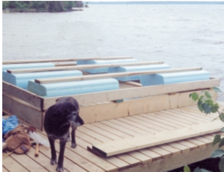
Dock under construction using untreated wood and blue polystyrene for flotation.
