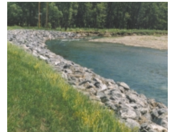
Bank stabilization using rock rubble.
