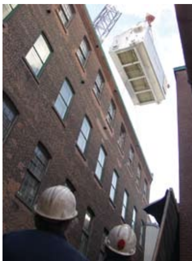
Installation of biogas energy unit at Cascades Fine Papers Group
