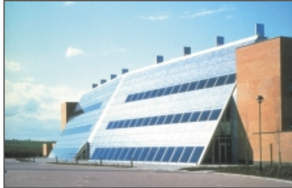
A 73 kW p PV array integrated into a 900 m 2 south facing façade inclined at 60 degrees, of the Solar Office at Doxford International Business Park, in England. The PV system is expected to provide 55,000 kWh of electrical energy per year, representing between one third and one quarter of the expected electrical usage of the building. (© Dennis Gilbert)
