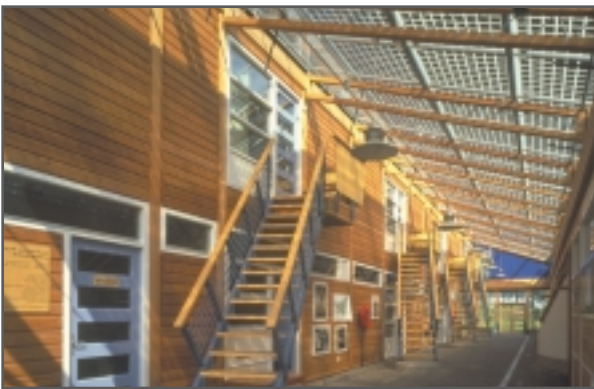
A glass corridor with integrated PV in an environmental education centre in the Netherlands. The solar modules combine two functions in one element, the produc- tion of electricity and shading, making this application attractive for many atria and sunspaces in large office buildings.
