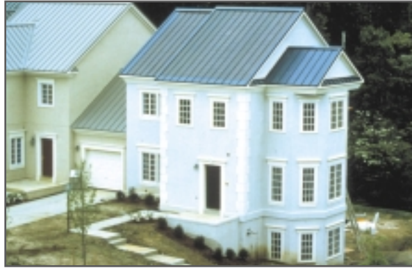
The UNI-SOLAR Architectural Standing Seam roofing system is used in an installation on a model 21 st Century Townhouse built by the National Association of Home Builders Research Center, Maryland, USA. The metal roofing module is identical to a standard seam and batten roofing plate. This system provides 1.5 kW and is grid-connected. All United Solar roofing products use the company's triple junction cell design. (© United Solar)
