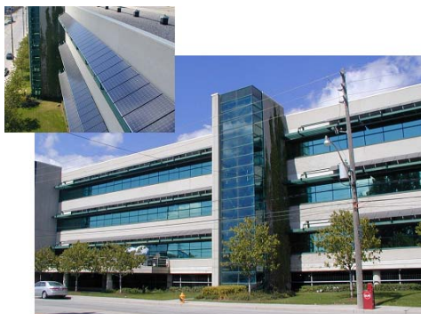
Figure 1: The Toronto Hydro Energy Services high-visibility pilot project in Downtown Toronto will generate 36 kilowatts of electricity. The provincial utility is providing Torontonians with an opportunity to see commercial installations in operation. (Photo credit: Phantom Electron Corporation)
