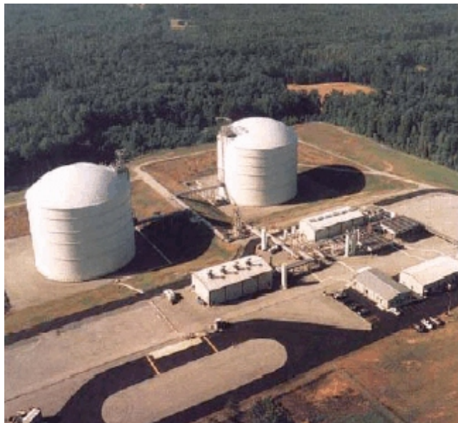
Peak-Shaving LNG Storage Facility
