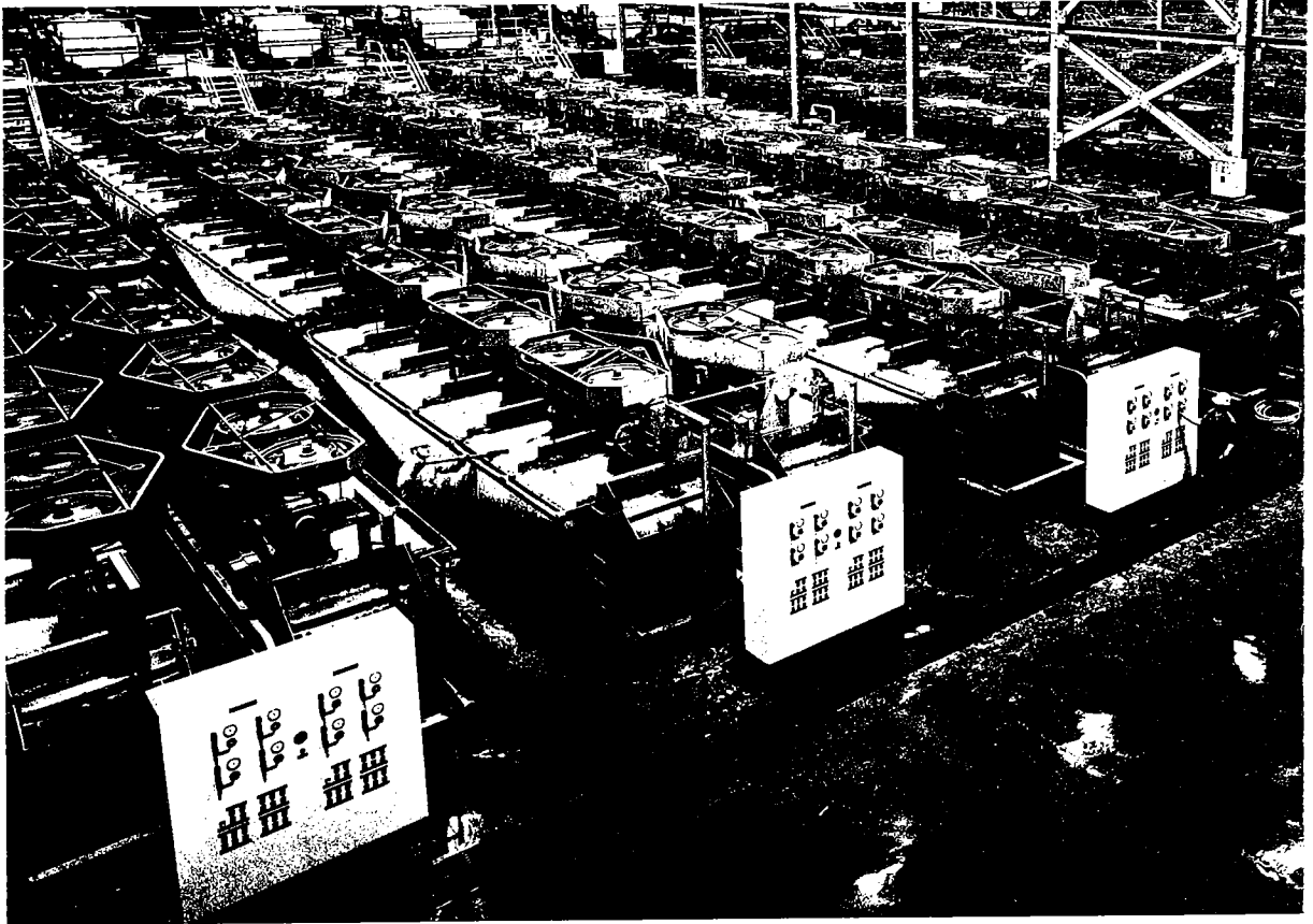
At Inco's Clarabelle Mill at Sudbury, Ontario, 528 flotation cells separate mineral particles from the rock waste through the action of chemical reagents. The panels in the foreground control this automatic operation. (Inco photo).
