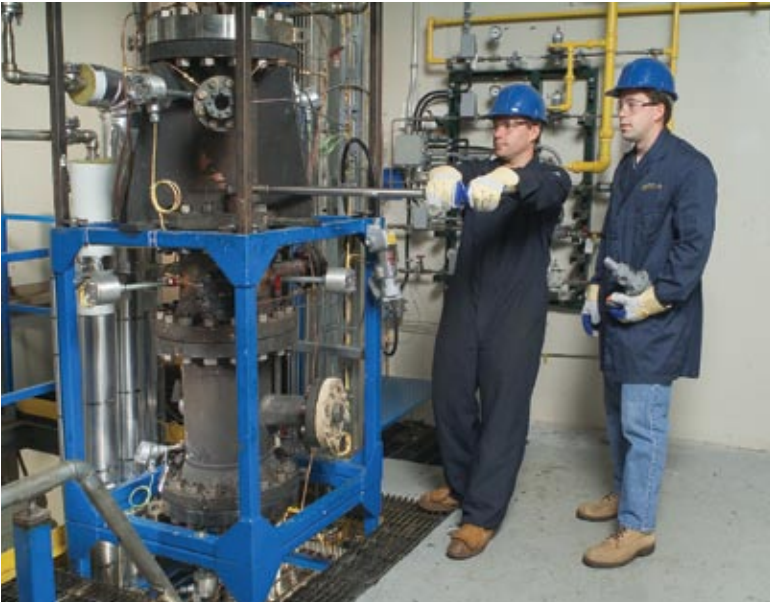
CETC – Ottawa is equipped with a variety of facilities and technologies to meet both industrial and commercial needs, such as this high-pressure gasifier, which produces a synthetic gas that can be used for producing hydrogen and clean coal power generation.
