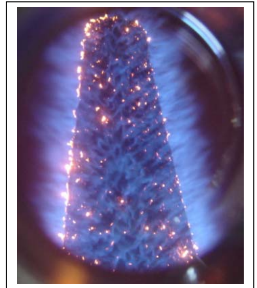
The micro-turbine duct burner operated in a blue flame mode
