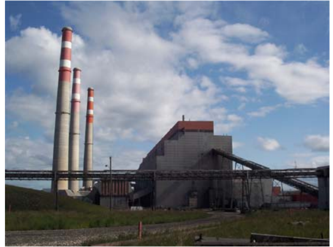
Coal-fired electricity generating station
