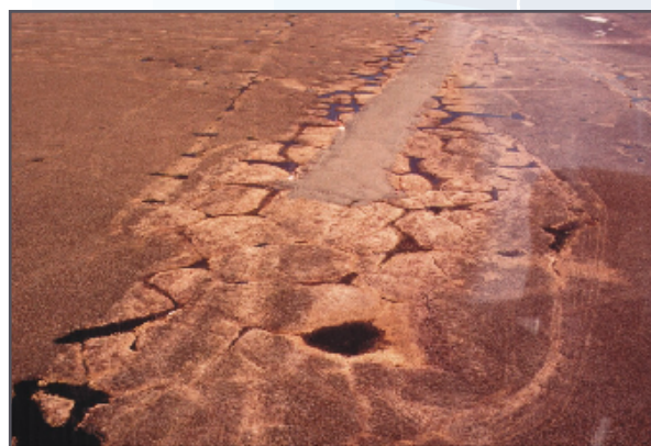
Degradation of polygonal ice wedges threatening the integrity of the abandoned airstrip at a DEW-line site.
