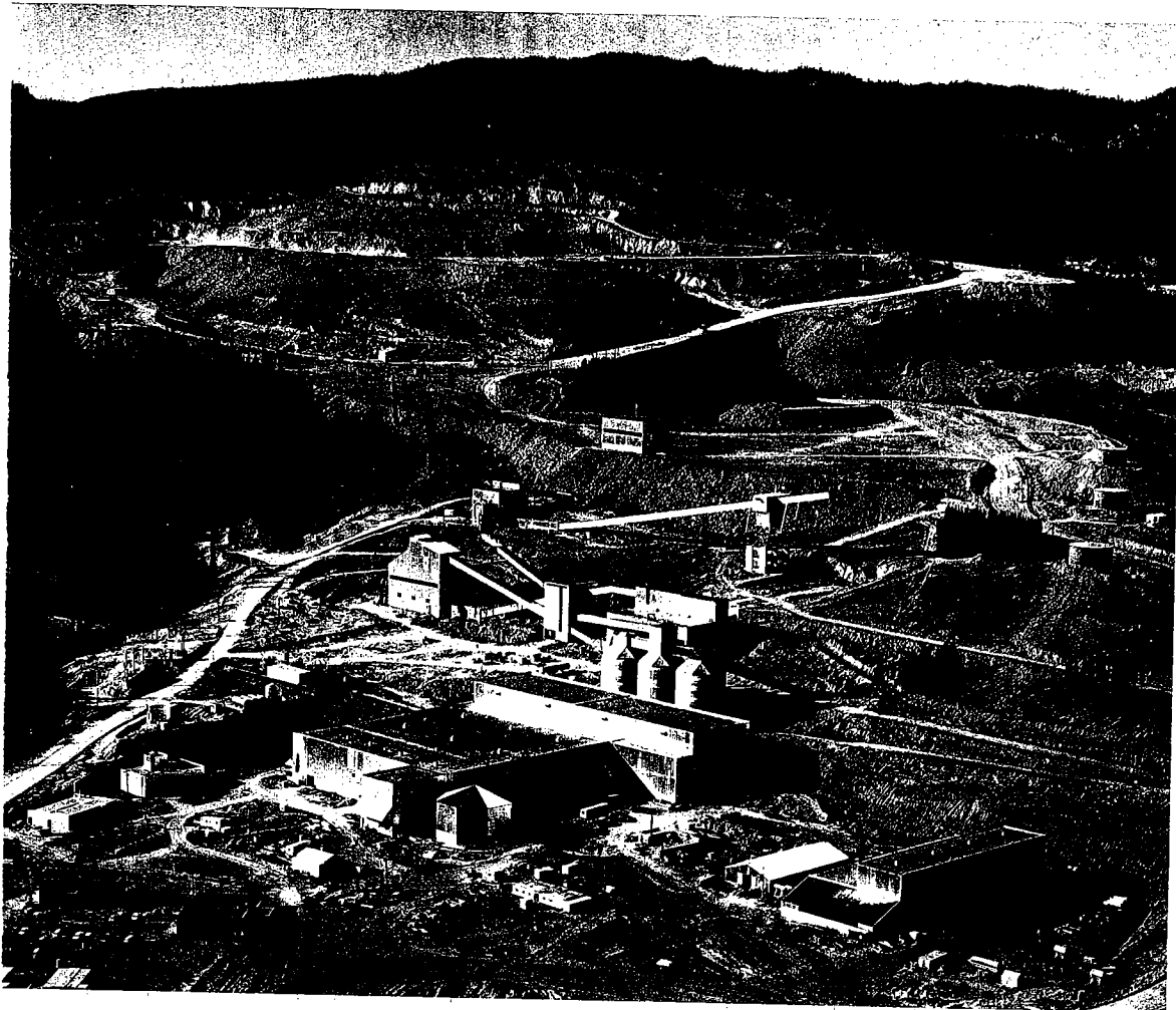
BRENDA MINES LTD, near Peachland, B.C. Open-pit preparation, upper left. Coarse crusher, upper centre. Secondary and tertiary crushing, fine ore bins and mill building, lower centre. Office building, lower left. Service bays, lower right. (Photo by Hunter)
