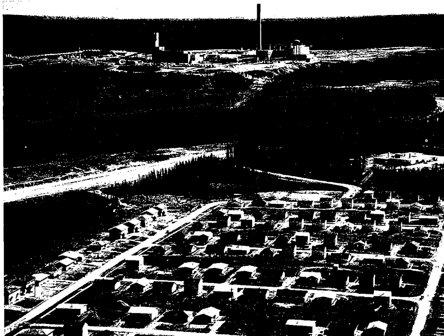
In north-central Manitoba, The International Nickel Company of Canada, Limited, started production in March 1961 from its giant Thompson nickel mine and refinery (above). By July, output was up to the rated annual capacity of 75 million pounds of nickel. Shipments of nickel to Europe were made through Churchill on Hudson Bay. Power for the electrolytic refinery and mine operations is supplied by the new Kelsey hydroelectric plant on nearby Nelson River (below).
