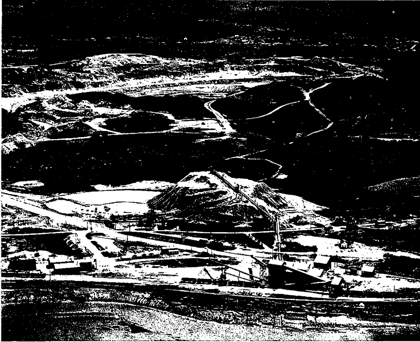
In central Nova Scotia, near Windsor, Canadian Gypsum Company Limited continued to produce gypsum, mainly for export to the United States for manufacture into plaster of paris and gypsum wallboard. In the photograph above, the quarry can be seen in the background, the waste dump in centre foreground and the mill and loading facilities in the foreground. The lower photograph shows the docks and storage facilities of the company at Hantsport, at low tide. During 1961, the Nova Scotia operations of the Company were taken over by Fundy Gypsum Company Limited. Nova Scotia produces about 85 per cent of Canada's gypsum production.
