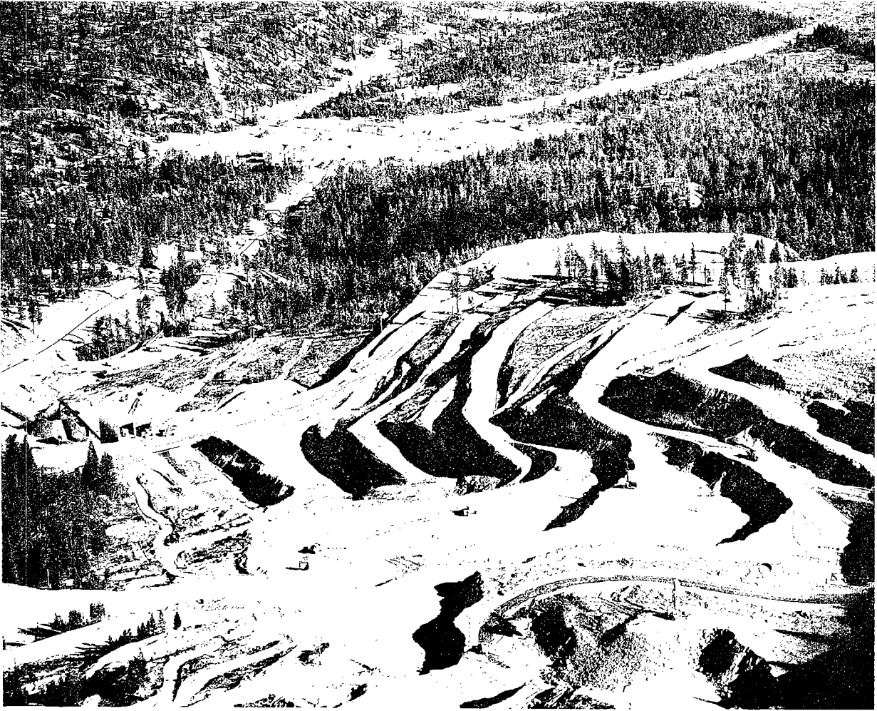
In south-central British Columbia, Craigmont Mines Limited began production from its copper mine. Ore from the open pit on the mountain slope (top) is trucked to a primary crusher and then carried on a one-mile cable belt to the mill and concentrator below (left). Concentrates are shipped to Japan and the United States.
