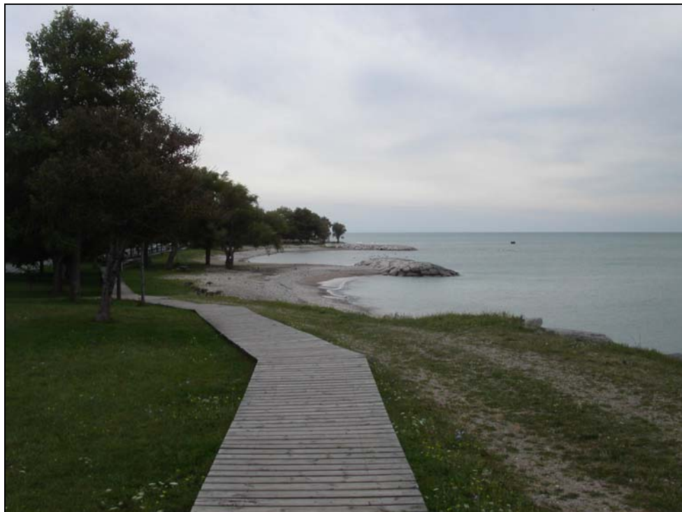
Figure 42: Goderich Harbour – Groynes Protecting Beach (M.Taylor).
