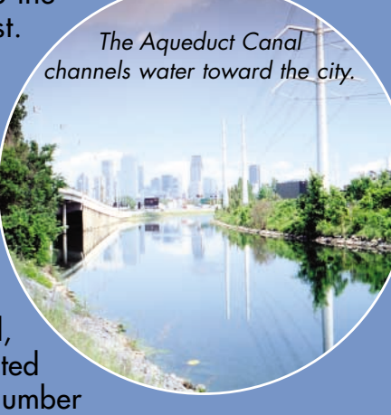
The Aqueeduct Canal channels water toward the city.
