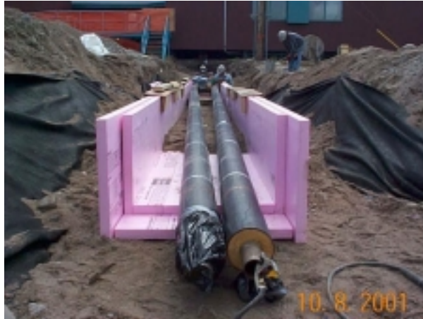
Piping trench between High School and Elementary School
