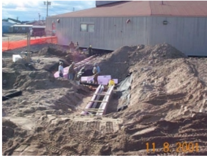
Piping trench crossing the schoolyard
