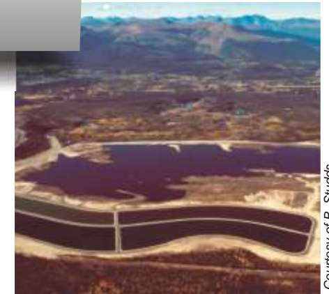
Treatment sewage lagoons and the one-year storage pond at Livingstone Trail Environmental Control Facility.
