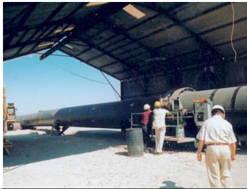
Summer 2002, Fusing of Pipe Belleville, ON on Bay of Quinte
