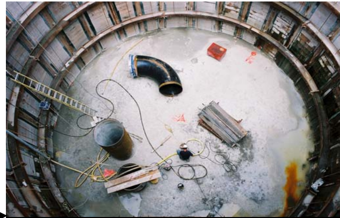
July 2003 Shaft Work
