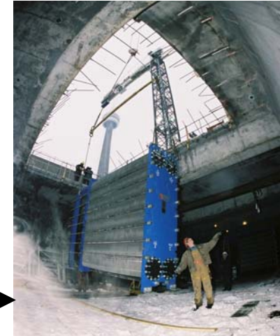
February 2004 Installation of HX
