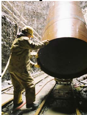
April 2003 Installation of Supply & Return Pipes
