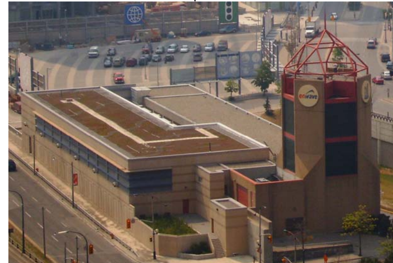
Summer 2004 Completed Energy Transfer Station
