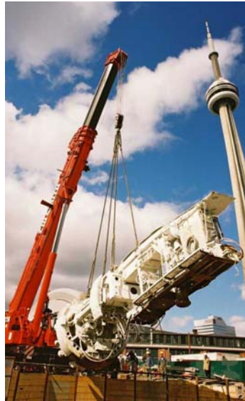
October 2002 Tunnel Boring Machine
