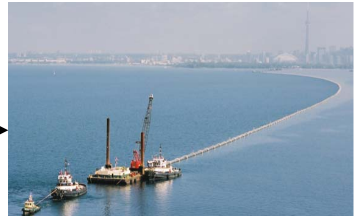
Summer 2003 –Deployment All 3 pipes in place by end of August 2003
