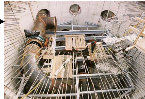
October 2003 Junction Valve Chamber
