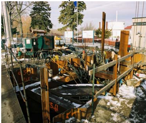
December 2002, Shaft Construction, Toronto Island
