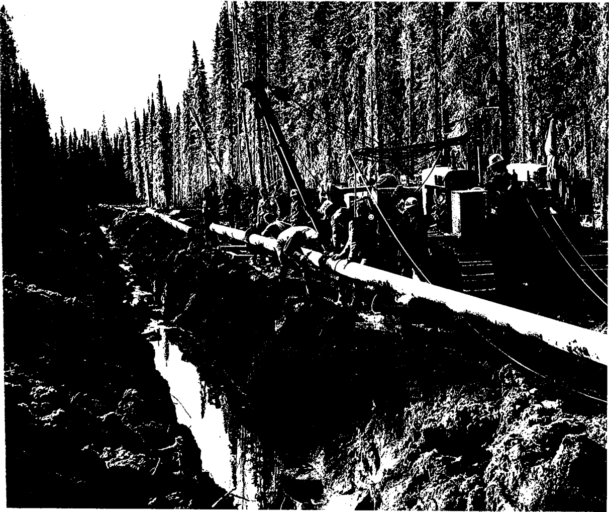
Installation of a natural gas gathering line in Alberta.
