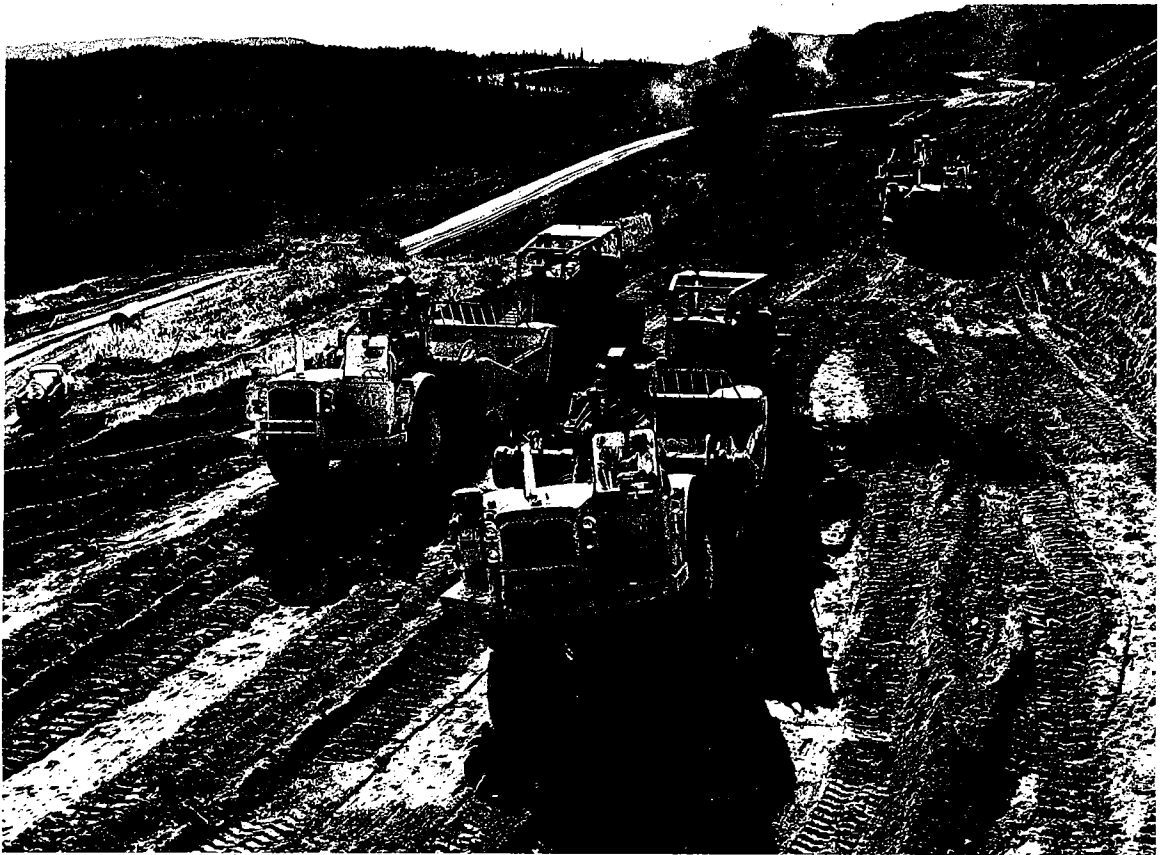
Stripping operations at the Endako mine.
